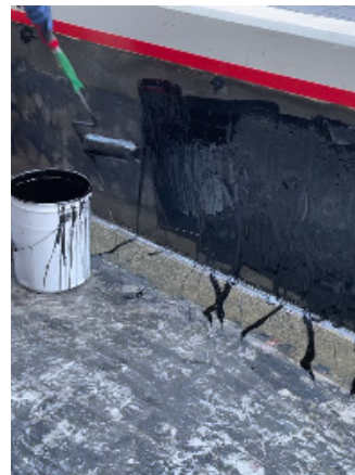
Step 2: Applied the vertical trowel grade to the wall and transitions
