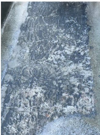
Step 1: Sandblasted the concrete & roughed up the surface to apply the primer
