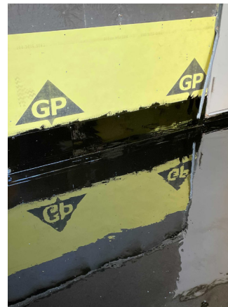
Step 3: Applied CIM 500 to waterproof the surface
