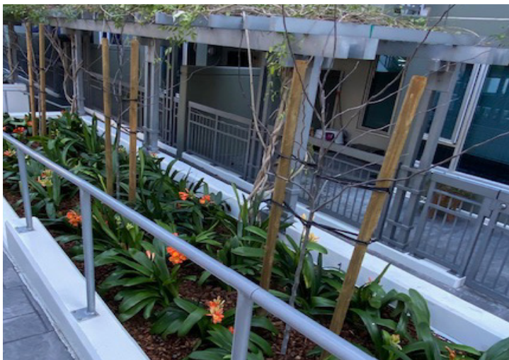
Image: CIM 500 waterproofing membrane applied on a concrete plant box
