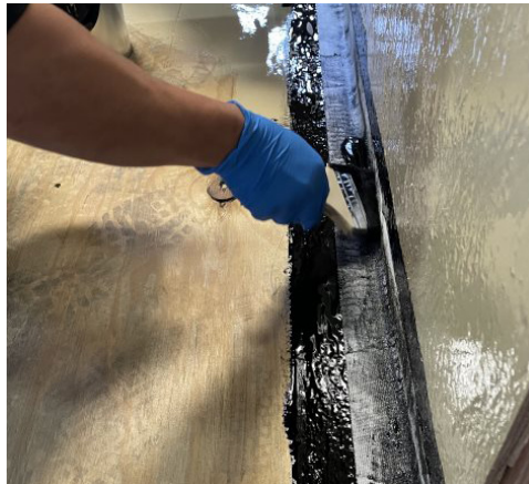
Image: Applying CIM waterproofing membrane
