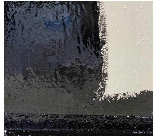
Image: CIM waterproofing (black) vs the ECO Epoxy Primer (tan)
